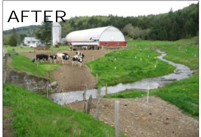
Installation of livestock fencing & buffer
