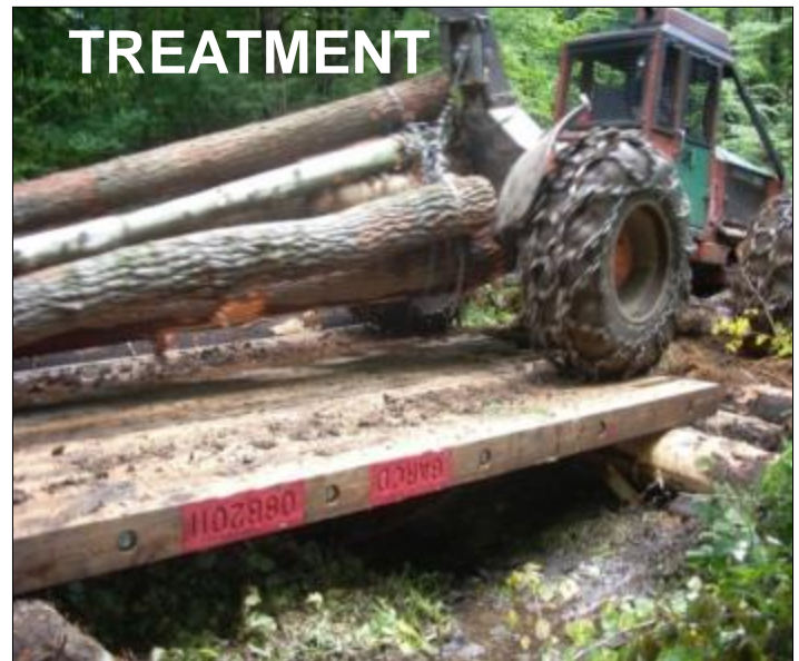
Temporary skidder bridge
